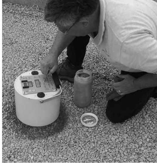
Figure 24. A base stiffness gauge can also be used to assess compacted density of aggregates.
