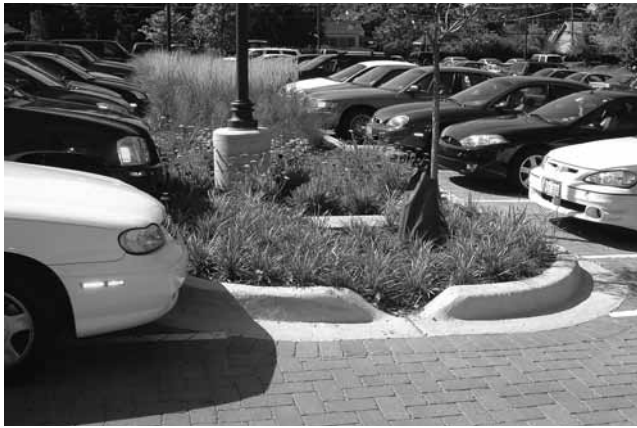
Figure 5. Elmhurst College, Elmhurst, Illinois parking lots uses full exfiltration through the soil subgrade with overflows directed through curb inlets into bioretention areas and overflow drains to manage extreme rain events.
