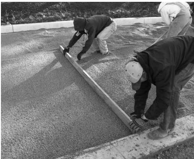
Figure 25. Manually screeding the No. 8 stone setting bed.
