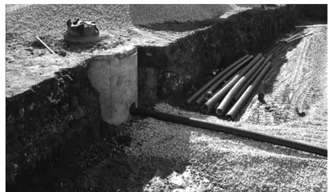
Figure 8. Partial exfiltration designs typically use perforated pipes raised above the soil subgrade. This enables capture and infiltration of some runoff.
