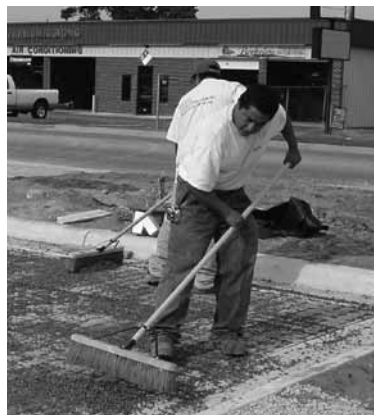
Figure 29. Various methods of filling and sweeping PICP joints.
