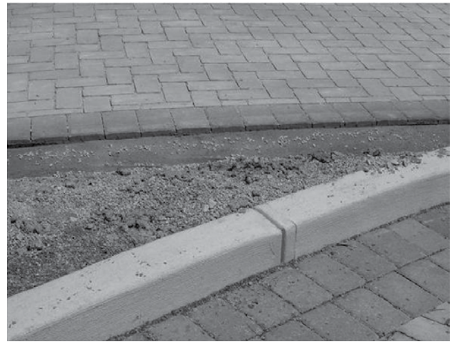
Figure 20. A PICP walk with a troweled concrete toe sits next to a driveway with a formed and cast-in-place concrete curb. Concrete toes should only be used for pedestrian applications.
