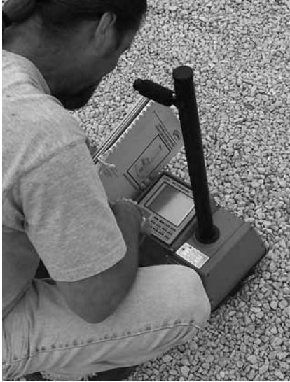
Figure 23. Density testing with a nuclear gauge in backscatter mode can help assess consistent density of the ASTM No. 57 base layer.
