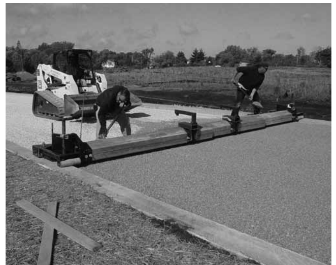
Figure 26. A screed beam pulled by equipment can be more efficient and productive.
